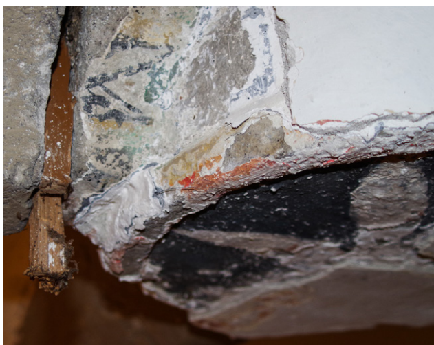
Detailed side view of the bolt; the remnant of the ornamental linear ochre-green painting is visible on part of the rib
