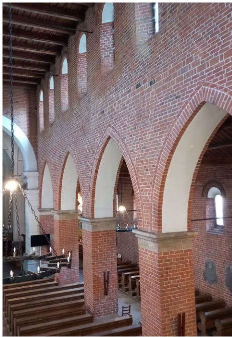
4. Southern inter-nave pillars (photo by M. Doroz-Turek, 2022)
