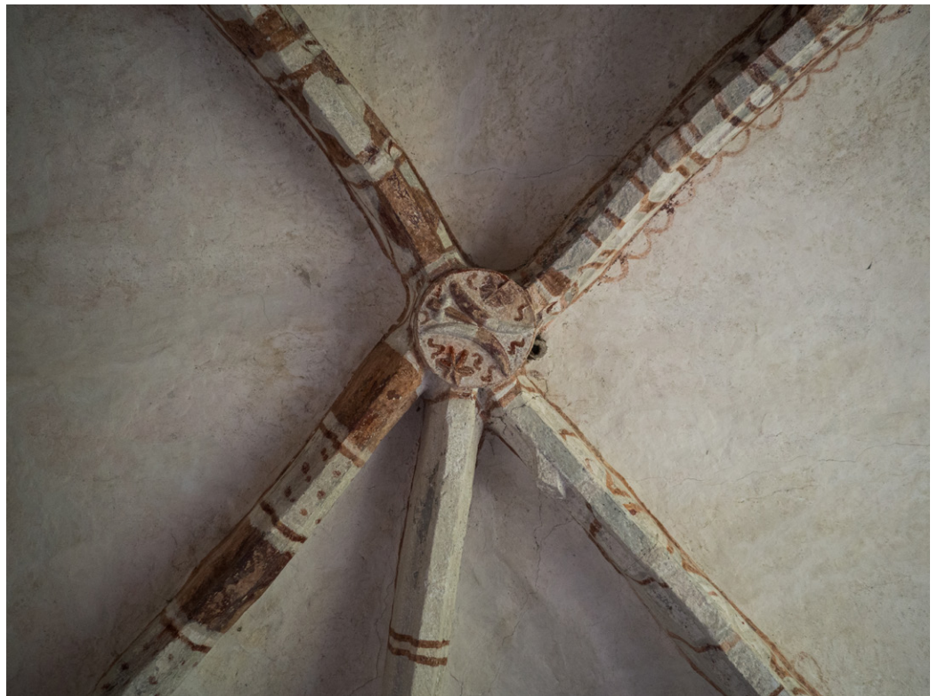
Rimavská Baňa (Rimabánya), sanctuary, keystone with Stibor coat of arms
