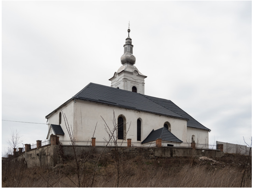
The Reformed Church in Rimavská Seč from the south-west
