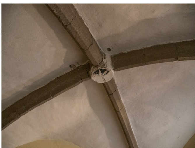
The view of the vault of the former sanctuary
